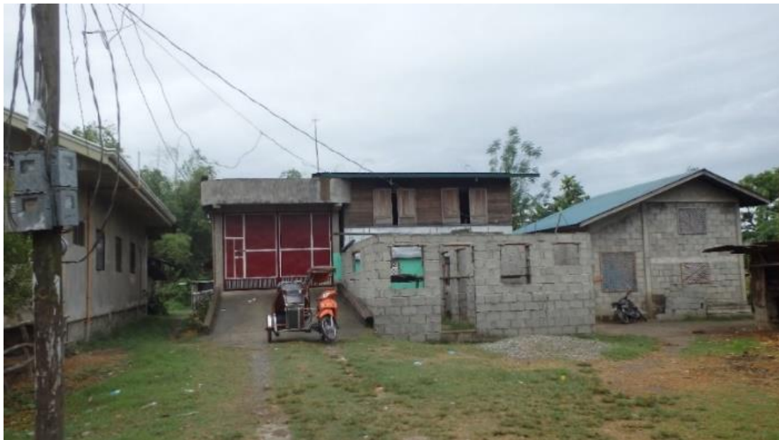
Figure VI. Elevated houses and establishment of 2 story houses
