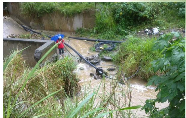
Figure 5. On-site setup of the hydraulic diaphragm pump
